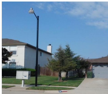
Light Poles are DONE!!!!!!
